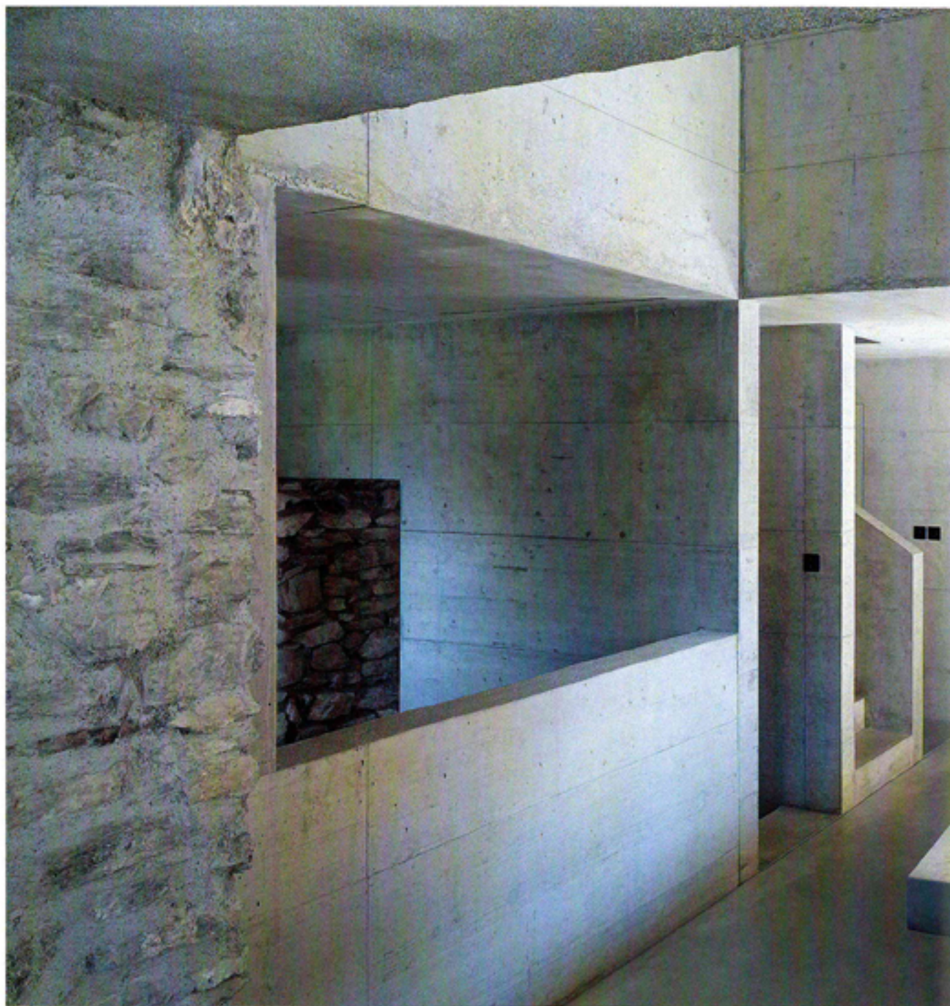
67 page: Interior view with old stone walls, exposed concrete and polished screed floors. p. 67, see: View of the atelier on 2nd floor (1) monolithic wall on the right. 7, below: View through kitchen and living room.
